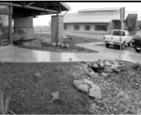
One of the most polluting aspects of developed land is the rain runoff from roofs and parking lots. When designing our new facilities, we included a dry creek system criss-crossing the lot. Rain water is directed into these creeks and allowed to filter through the rock and soil before draining into the gutters or naturally into the native creek off the back of our parking lot.
