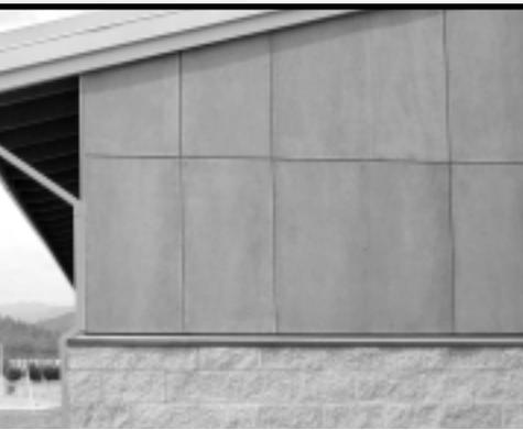
The exterior walls of each of our buildings are covered in concrete fiber panels. Not only are they constructed of recycled materials that are relatively clean to manufacture, but they are also weather resistant and require no paints. Finally, they are mounted on a vertically orientated frame creating convection cells that function to reduce radiant heat gain to our building.
